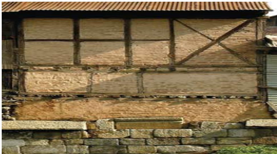
Fig.2: Showing elevation of Dhajji-Dewari Construction in Down-Town Srinagar
