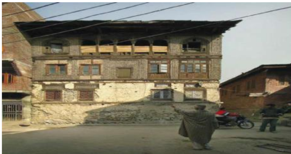
Fig.1:Showing Taq construction in Srinagar
