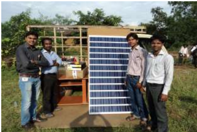
Fig - 2.4 : Solar power system
