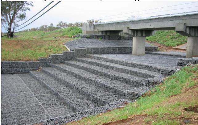
**Fig -4:** An Apron of Gabion, protecting the stream bed from being scoured.
