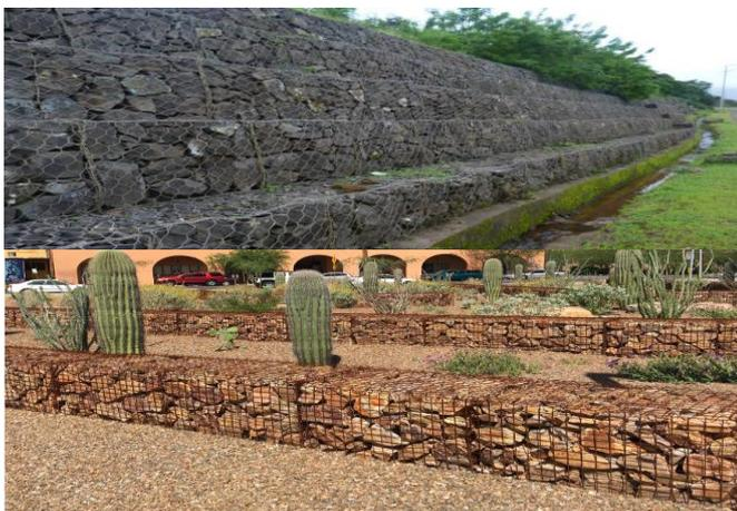
Fig -2: Hexagonal mesh (top), square mesh (bottom).
