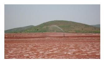
Figure 4.Sprinkling system of red mud pond to prevent dust effect at Damanjodi
