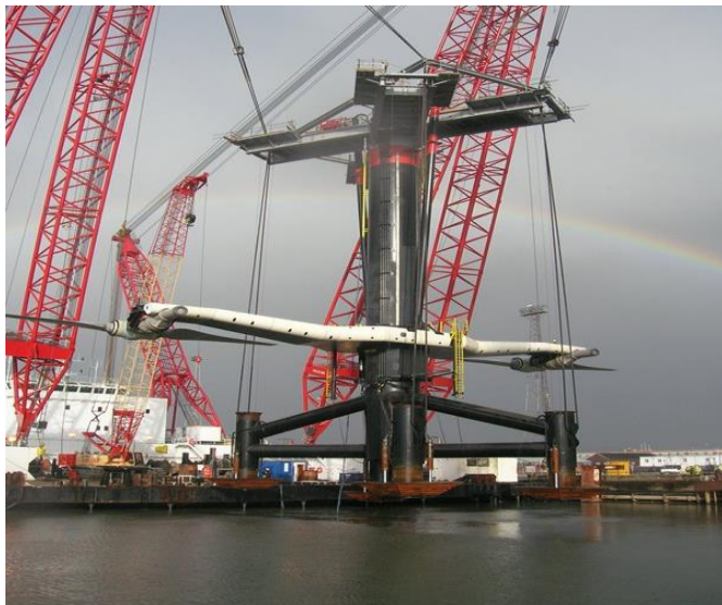
Fig.14. Installation of Seagen.
