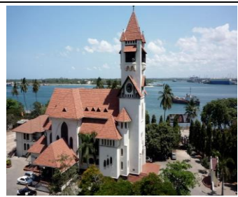
Fig-4.4: Azania Front Lutheran Cathedral is "Christian Church under the Eastern and coastal Diocese of the evangelical Lutheran Church in Tanzania". Constructed in Gothic style between 1899 and 1902.
