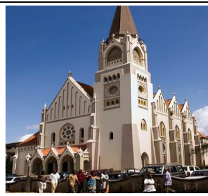
Fig-4.3: St. Joseph Catholic Cathedral is "Christian church". Constructed in Gothic style by the Germany missionaries 1889. Stands magnificently along the kivukoni road.
