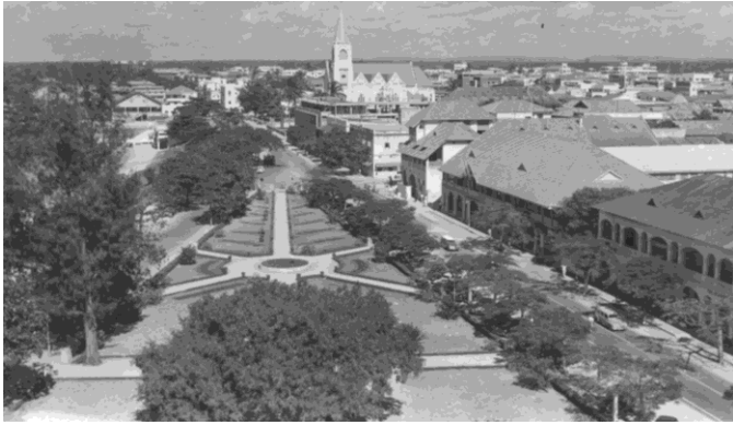
Fig. 6.1: An aerial view of Dar es Salaam's skyline in which the Saint Joseph Cathedral church in stable communities was the only building at the centre which rose high above the surrounding built fabric. The buildings that preceded it (right) maintained a uniform skyline ranging between 2 and 3 storeys. (Source: DCC).
