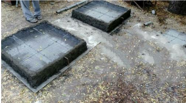
Fig-3: Box Like Structure
