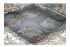
Fig3.4: Column Center Line Marking
