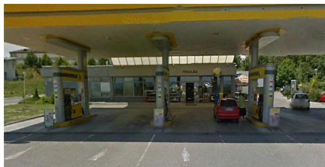
Figure 2: Overall situation at the petrol station
