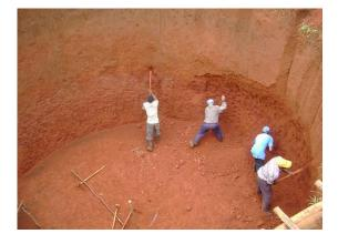
Fig -4 Pit of Bio Gas chamber. STEP 4: Installation of digester bag
