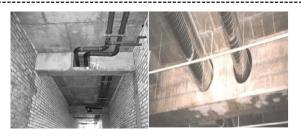
Fig 1.1; RC Beam with opening
