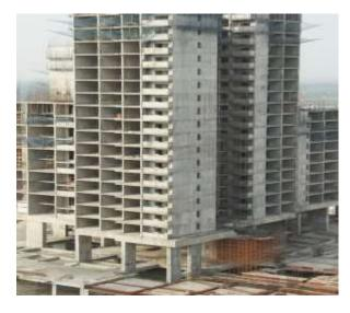
Fig 1. Transfer slab
