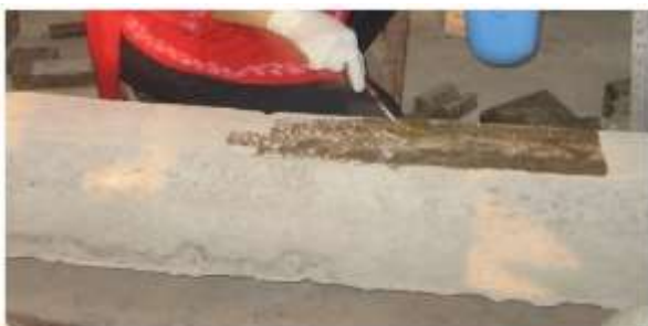
Fig.-3: Usage of Epoxy and hardener on the beam
