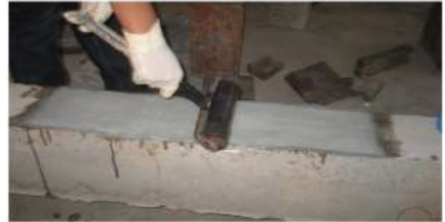
Fig.-4: Roller used for the removal of air bubble
