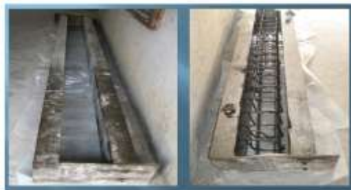
Fig.-2: Steel frame utilized for casting of beam
