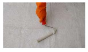
Fig 8: Removal of air bubbles using roller
