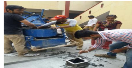
Fig 2 Mixing of Concrete ingredients using Pan Mixer
