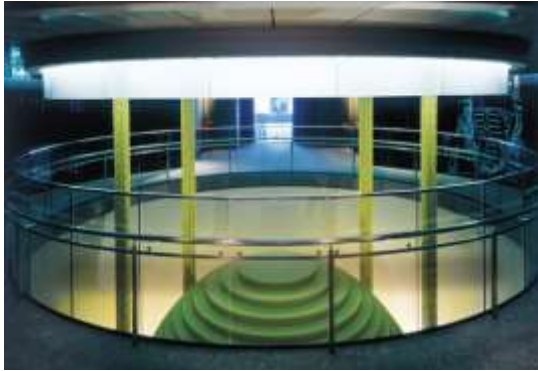
Fig -2: Tuned Mass Damper in Taipei 101
