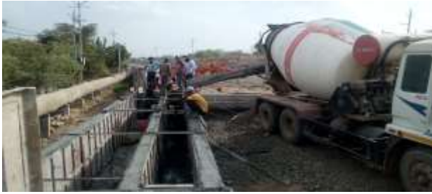
Fig -1: Discharging of RMC at project Site
