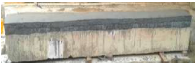
Fig -7 Repaired Damaged Beam
