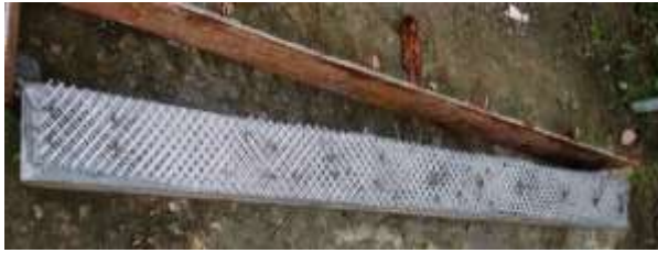
Fig -5 Repaired Damaged Beam (steel mesh at 45°)
