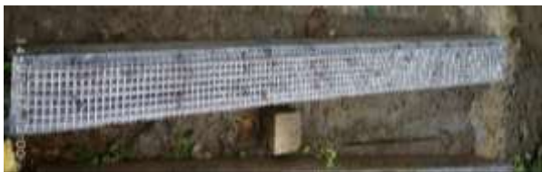
Fig -6 Repaired Damaged Beam (steel mesh at 90°)
