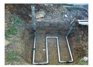
Fig. 1 Actual Set up Of EATHE system
