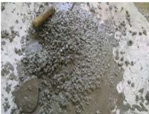
Figure12 Mixing concrete with Fibre
