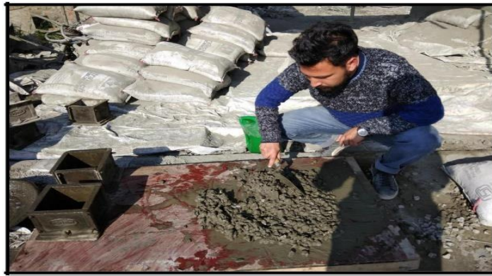
Figure 7. Hand Mixing of Concrete
