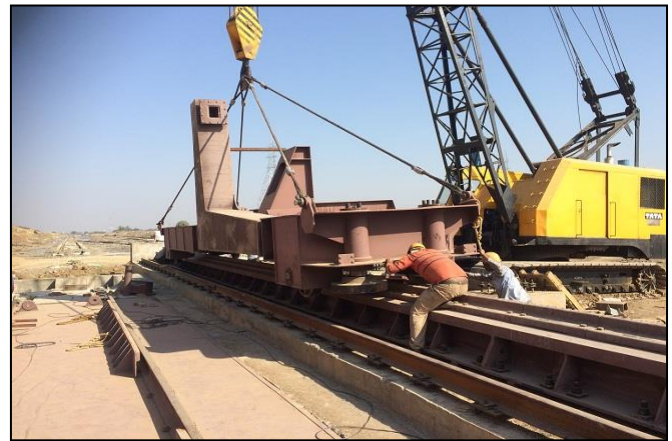
Figure-13: Erection of the Side arm charger
