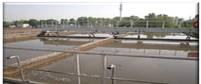
(Primary settling tank of wastewater treatment plant)
