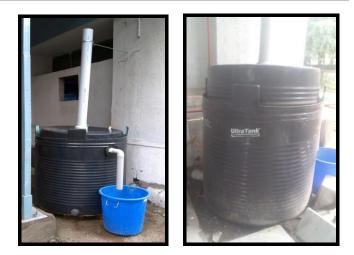
Fig-2: Biogas plant from canteen kitchen waste in A. C. Patil College of Engineering, Kharghar, Navi Mumbai
