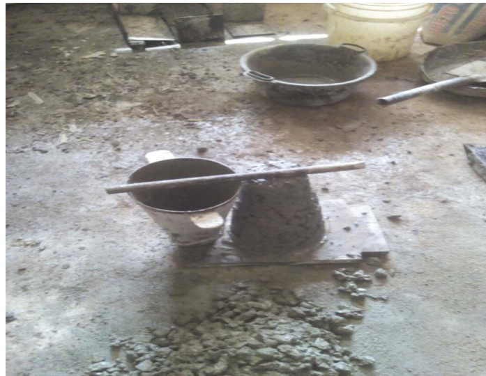
Plate 1: Slump Test for the Concrete mix
