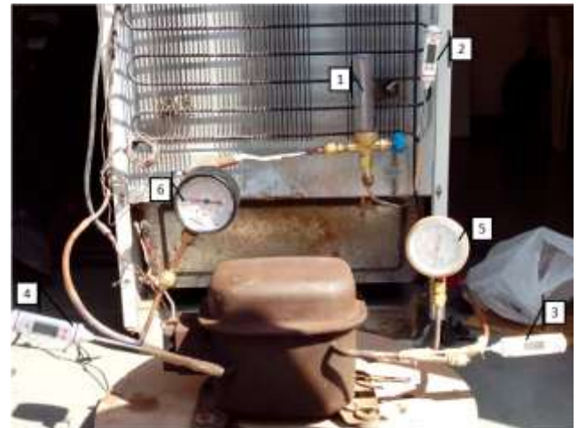
Fig -1: Arrangement for finding out amount of heat ejected by condenser of household refrigerator [1- flow meter, 2,3,4 - Digital temperature sensors, 5,6 - Pressure gauges]
