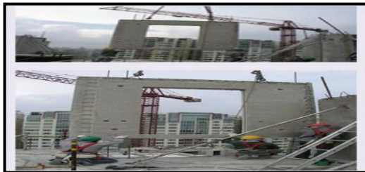
Fig-6: Lifting & Adjusting the components
