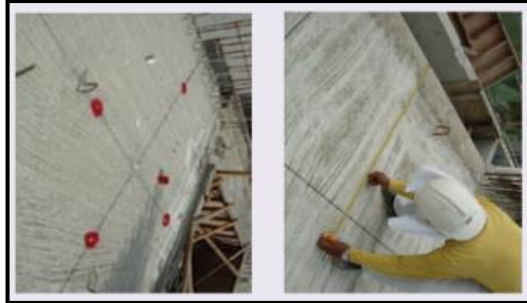
Fig-9: Marking of Reference Line
