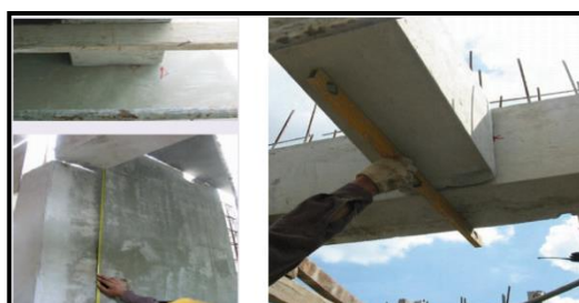
Fig-11: Align and Check Level
