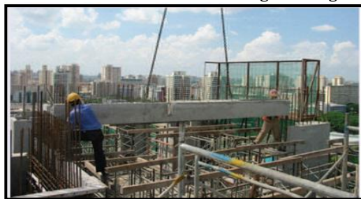
Fig-10: Lifting and Temporary props
