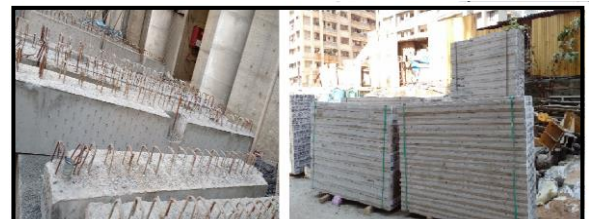
Fig-3: Precast Beam
