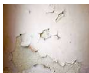
Photo -1: Visual Inspection of Cracks and Damages of Plaster in Building.
