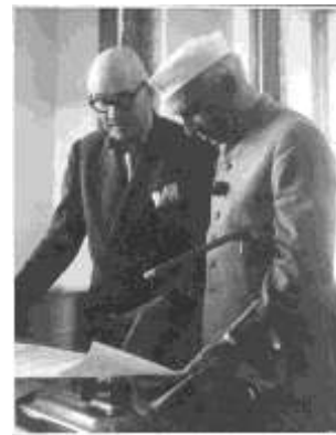
Fig -2: Interaction between Nehru and Le Corbusier (Source: Fondation Le Corbusier, Doc. L4-3-6)
