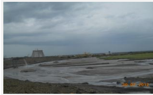
Fig. 4: Disposal of Pond Ash
