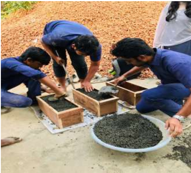
Fig 3. Casting of solid blocks
