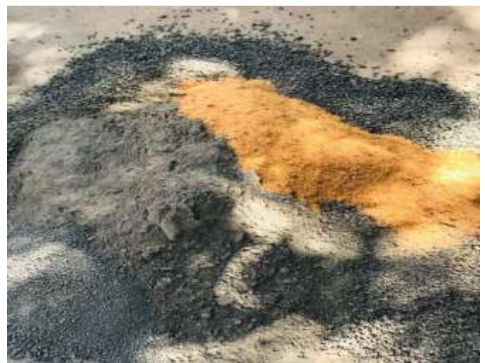
Fig 2. Dry mix for casting of solid blocks
