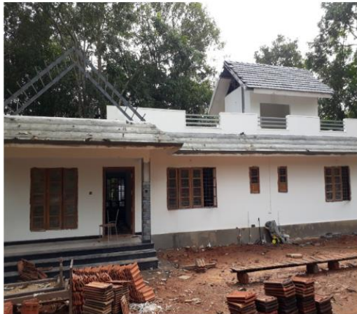
Fig 2:- Building at Chalakudy, Kerala
