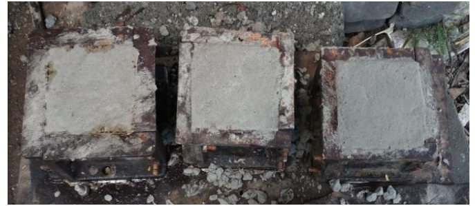
Fig -2: Casting of Cube
