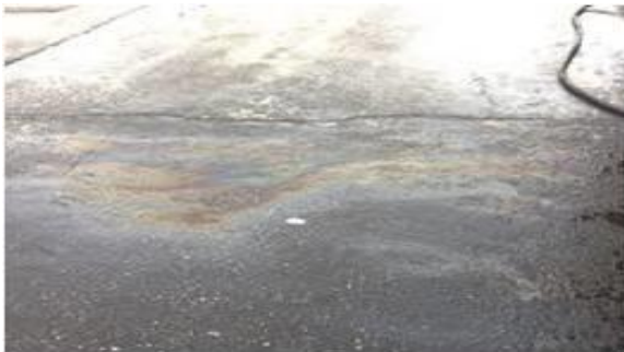
Fig -2: Flow of Mixed Acid on Concrete
