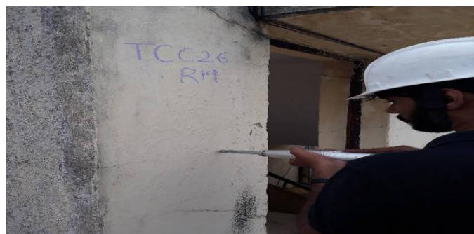
Fig -1: Rebound Hammer Test
