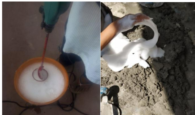
Fig -1: Foam preparation and mixing of it by prefoaming method
