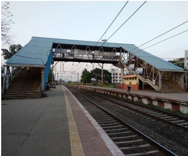
Fig -1: Rcc foot over bridge at shelu station
