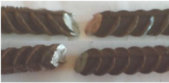
Fig -4: Failure of steel bar
