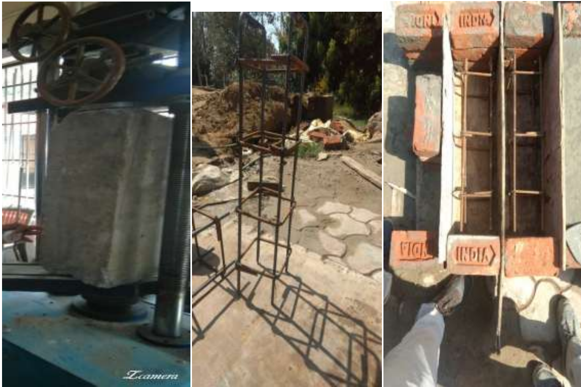
COLUMN TESTING ON UTM Reinforcement of column Casting of Column
