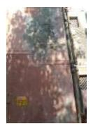
Fig -10: Flaking of plaster
