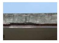
Fig -8: Deterioration of cover
