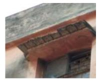
Fig -9: Failure of chajja
