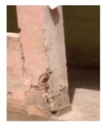
Fig -5: Cracks in Column
