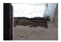
Fig -6: Spalling of concrete
