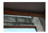
Fig -4: Flexural Cracks in Beam
