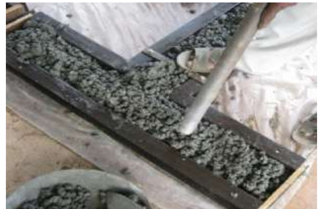
Fig- 3: Casting of control specimens (CS)
