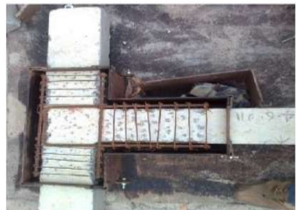
Fig-4: Casting of retrofitted specimen
