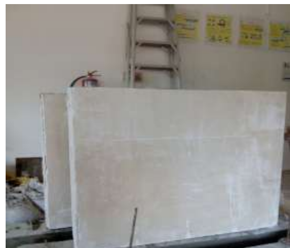
Fig-5: Placing of panel above plinth beam
