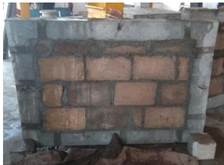
Fig- 3 Frame infilled with MCB
