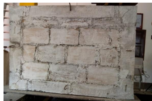
Fig-6 Crack Pattern
