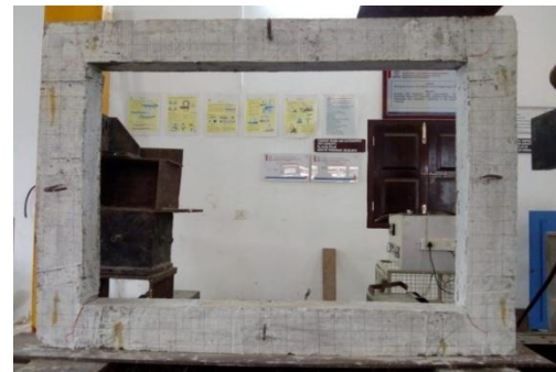
Fig- 5 Crack Pattern
