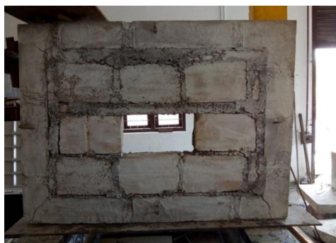
Fig-7 Crack Pattern
