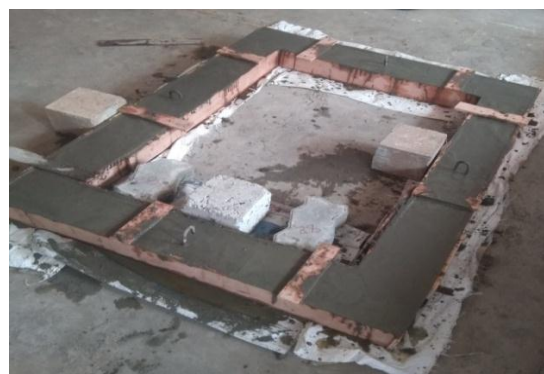
Fig-1 Casting of RC Frame
