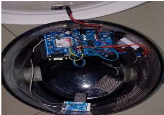
Figure 2. Top view of manhole attached to the sensors
