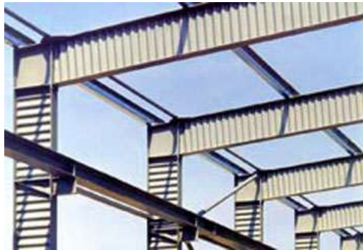
Fig - 1 Corrugated Web Beam
