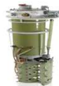
Fig -10 Vacuum type tap changer(ABB)
