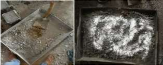
Fig 3.1- Mixing of concrete with Nano-silica
