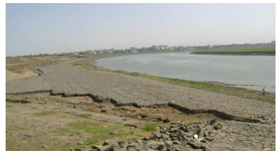
FIG 7- River bank protection
