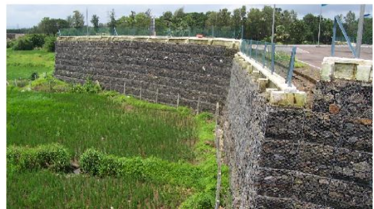
FIG 6- Gabion retaining wall
