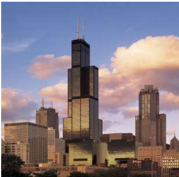
Figure 2: Tube Structural Design Tower
