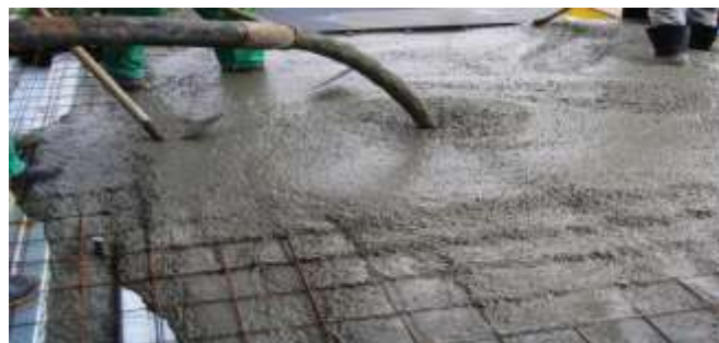
Figure 1: Self-compacting concrete using in slab
